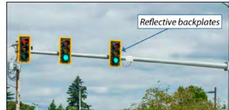
*Safety improvements include installing reflective backplates on traffic signal heads and upgrading existing signs for better visibility.*
